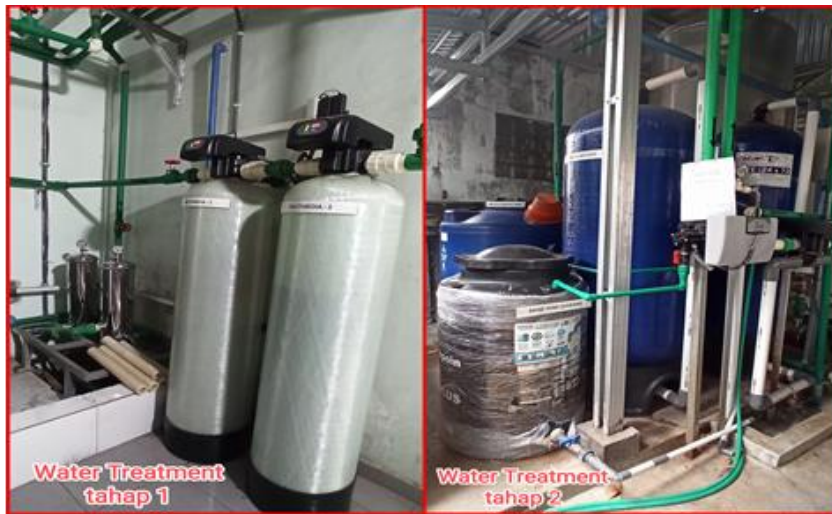
Gambar 4.4 Sistem Water Treatment
