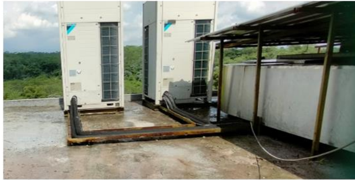
Pencucian HVAC Kamar Operasi
